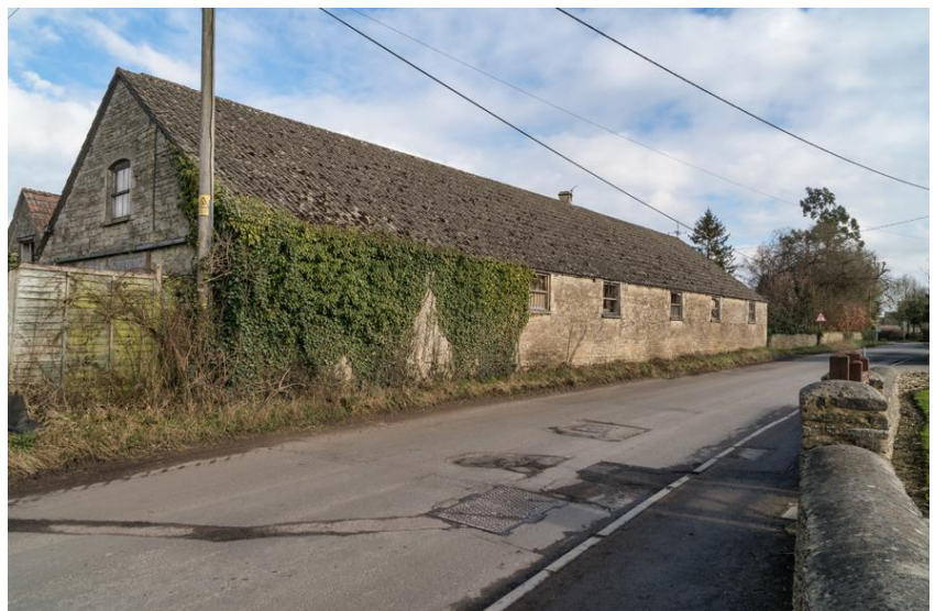
Barn at Street Farm, The Street
