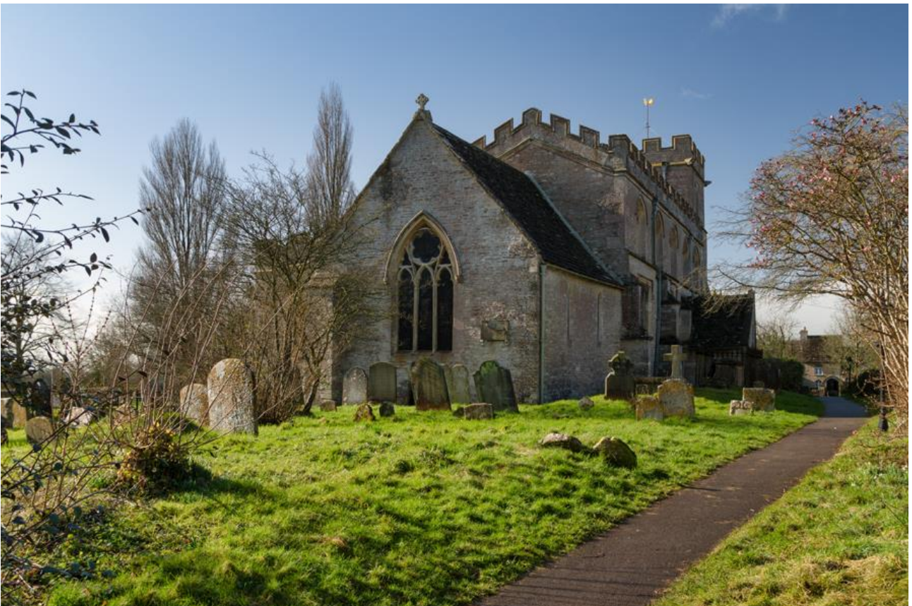
Church and Footpath Looking West
