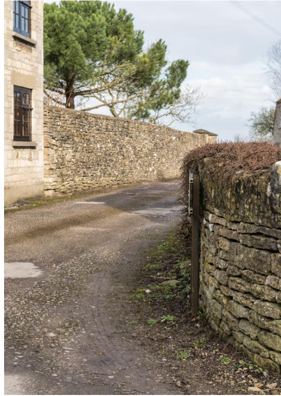
Stone Walls, Coppice Lane
