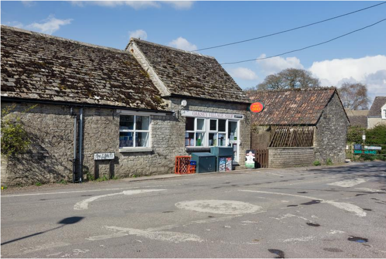
Shop and Post Office (Former Butchery and Abattoir)
