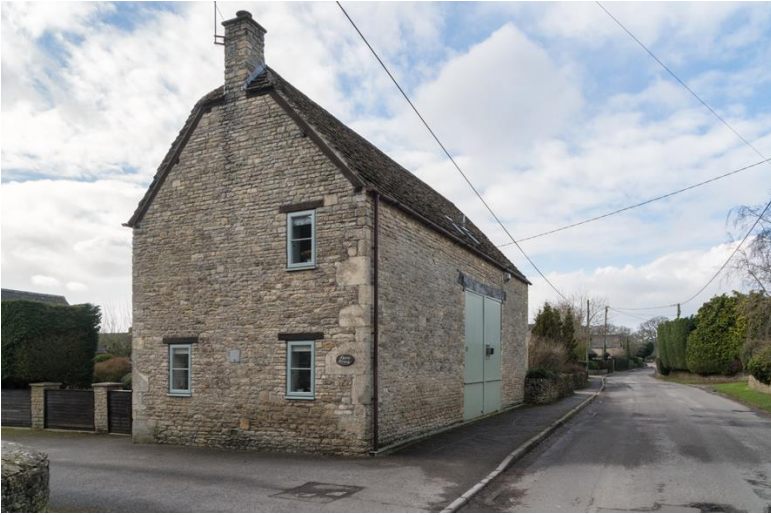
Barn House, South Street
