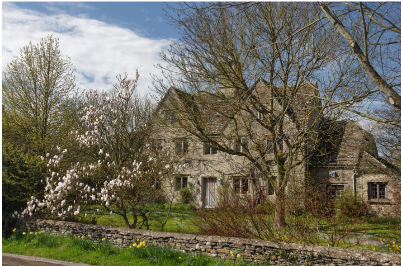
The Old House on The Corner of The Street and Wheatsheaf Lane
