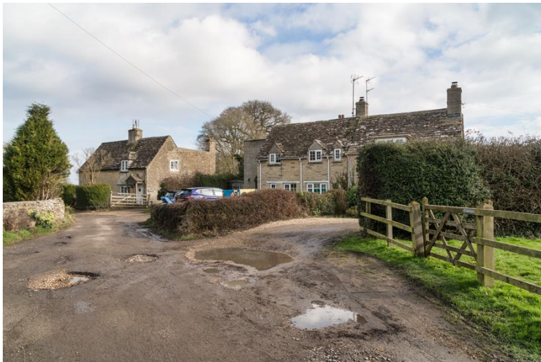
Cottages on Earls Corner
