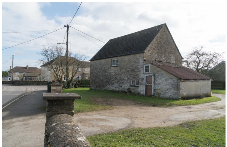
Barn Adjacent to Junction with The Green
